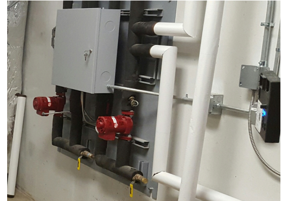
Factory-built TRICOIL pump pack on a 36 × 48 in. wall panel: loop and heating pumps, control valves and prewired controls.
